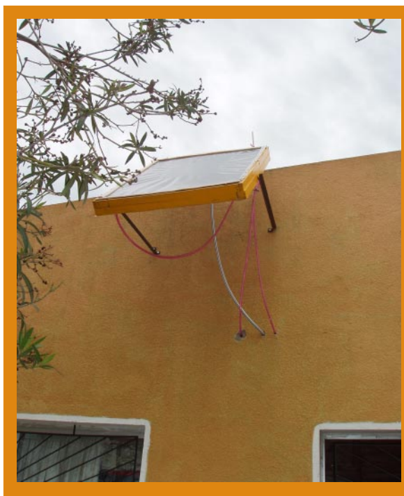
Calentador solar autoconstruido, LaTAs, Liceo de Baltasar Brum, departamento de Artigas / Self constructed solar heater in Baltasar Brum High School, Artigas department - Foto: UCC - DINAMA
